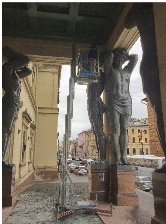
Fig. 1. Laser scanning process
